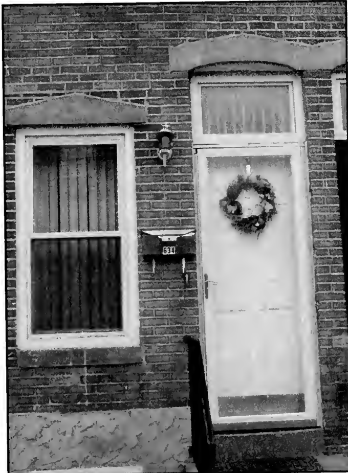
Figure 7: Cast concrete replacement details. Photo taken by Amy Simcik, 2003.
